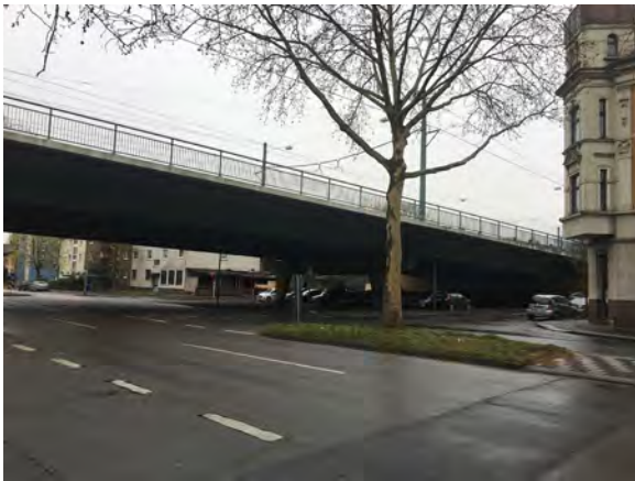
Figure 08 - Berliner Brücke saw from below (2019)
