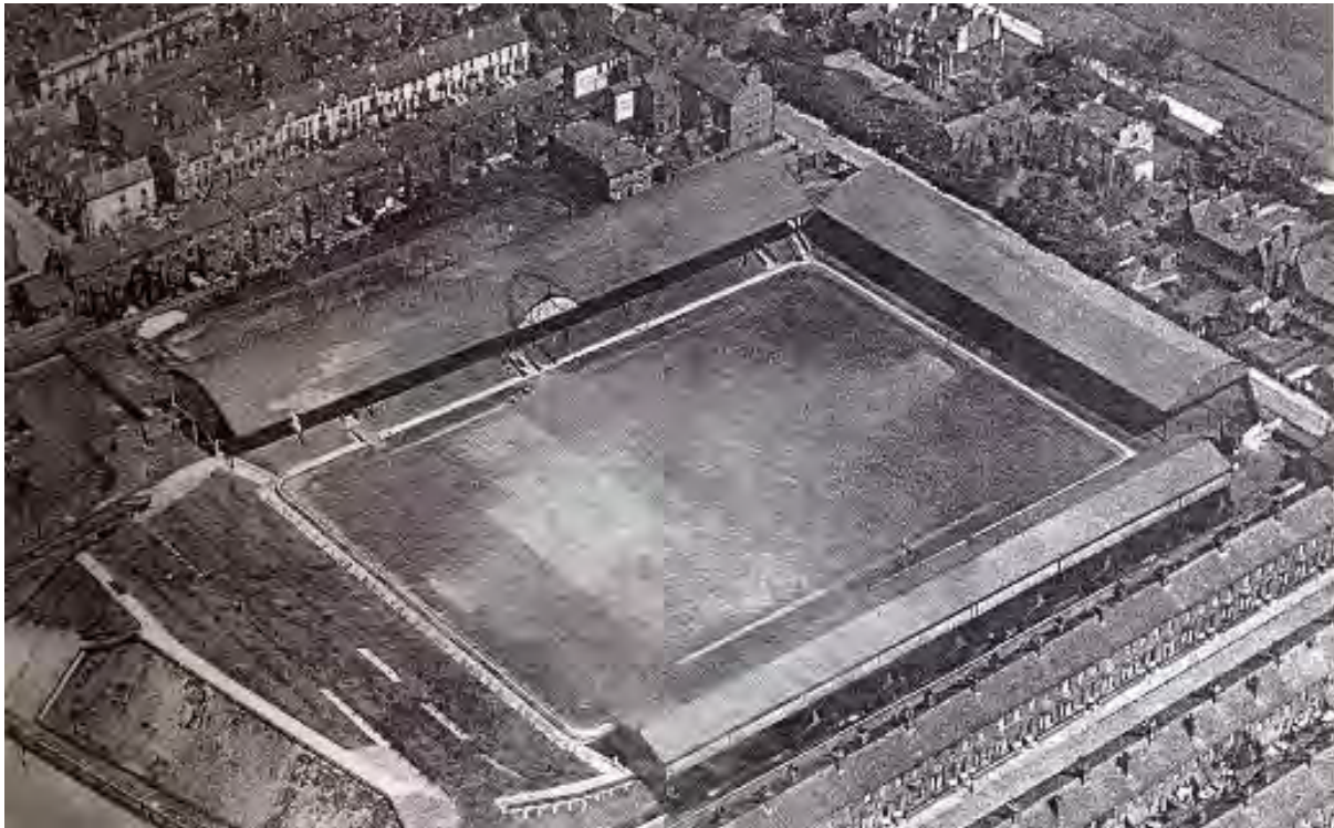
Figure 13: Anfield Stadium in the 1920s (source: stadiumguide n.y.)
